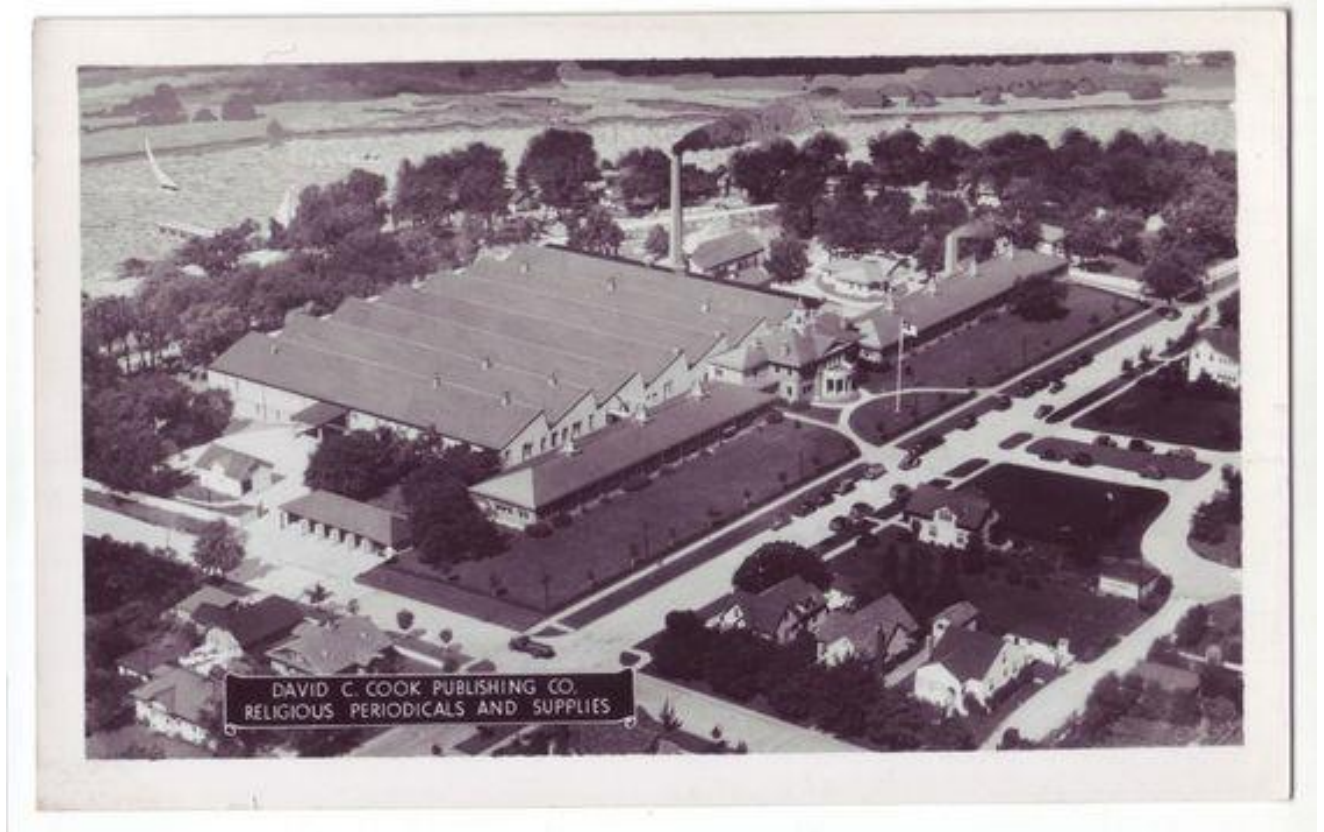
Figure 6: Aerial View of D. C. Cook Publishing House
